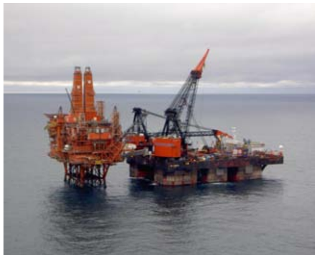
North West Hutton decommissioning (removal) with lift barge alongside
