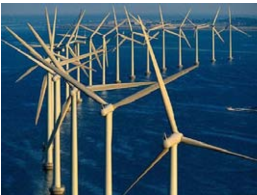
Offshore Wind Farms – will the subsea component of such structures – like many wrecks - form new marine colonies over time?
